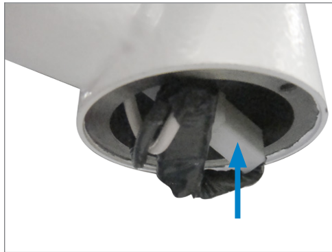
Connect Cables and push them up
