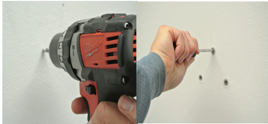
Figure 7-3 Drill and Prepare Mounting Holes
