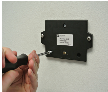
Figure 7-4 Attach SmartBracket to Wall
